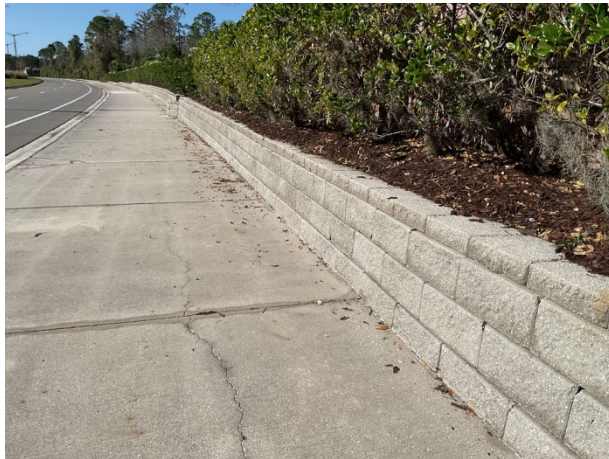
Masonry retaining wall at Capri at La Vina
