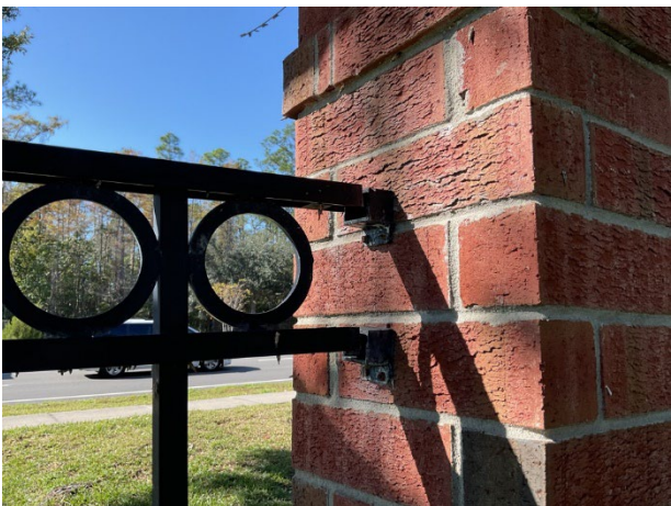
Fence detached components at Lake Nona Preserve
