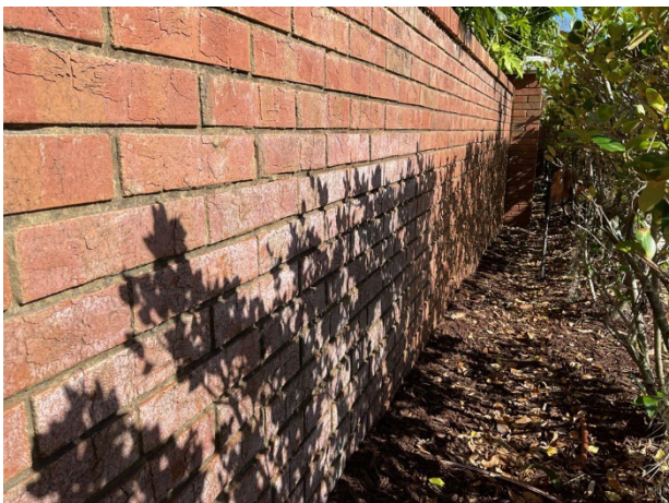
Wall efflorescence at Capri at La Vina
