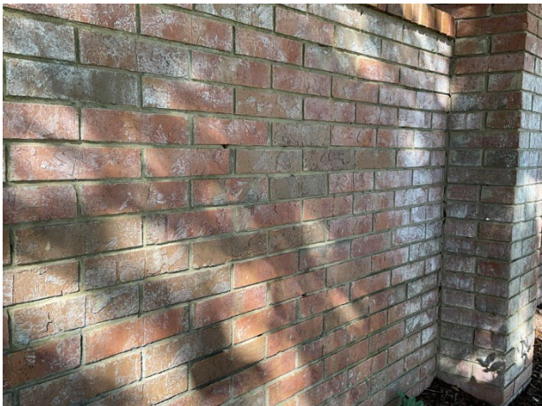
Wall mortar deterioration at Mirabella at La Vina
