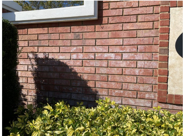
Efflorescence at Capri at La Vina entrance monument
