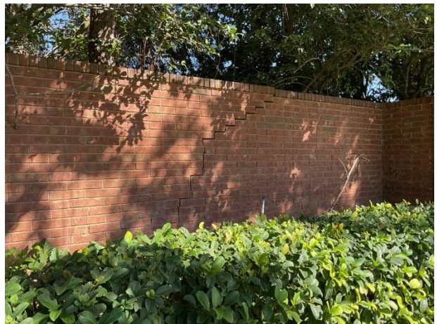
Wall cracks at Nona Crest perimeter
