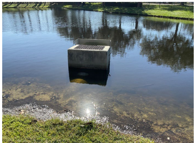
Pond control structure at Lake Nona Preserve
