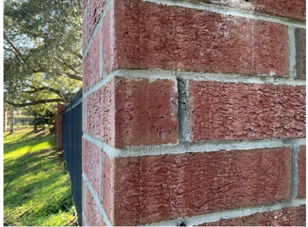
Wall mortar deterioration at Lake Nona Preserve
