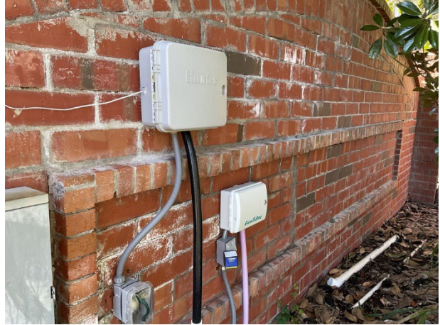
Irrigation system controllers at Lake Nona Preserve entrance monument
