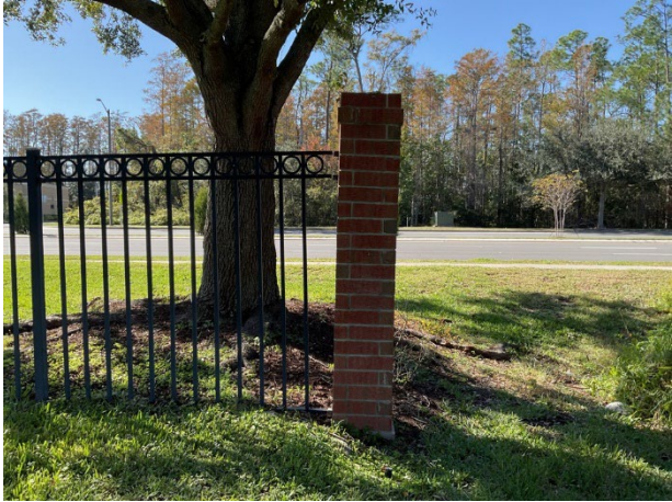
Leaning masonry column at Lake Nona Preserve west perimeter
