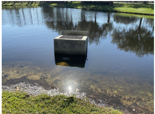
Pond control structure at Lake Nona Preserve
