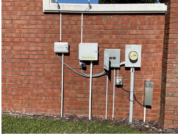
Irrigation system controllers at Ziani at La Vina entrance monument
