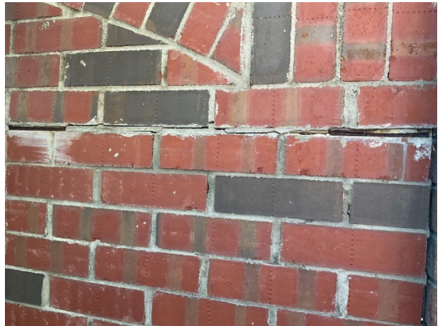
Wall mortar deterioration with exposed reinforcement at Lake Nona Preserve entrance monument
