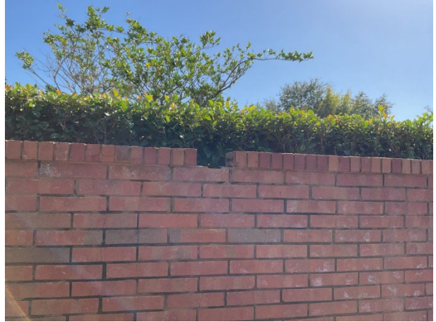
Missing masonry at Ziani at La Vina
