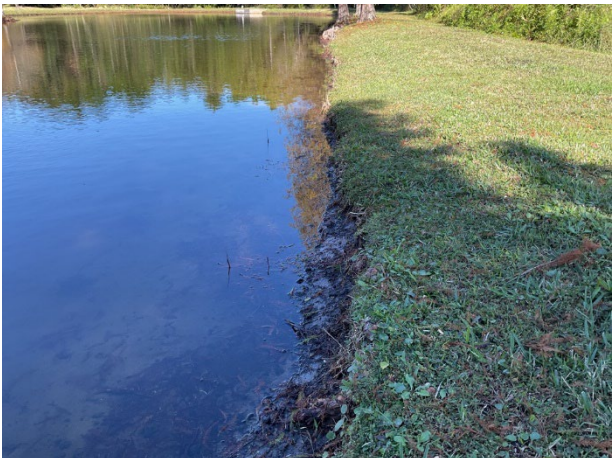
Erosion at Lake Nona Preserve tract H
