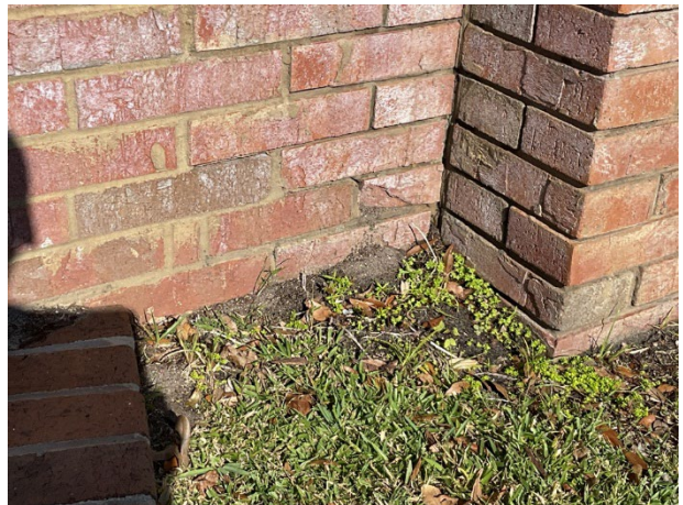
Wall brick spalls at Mirabella at La Vina
