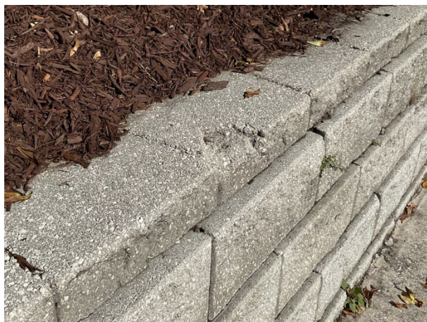
Spalled masonry
