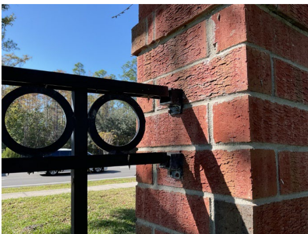
Fence detached components at Lake Nona Preserve
