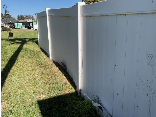
Fence leaning section at Nona Crest
