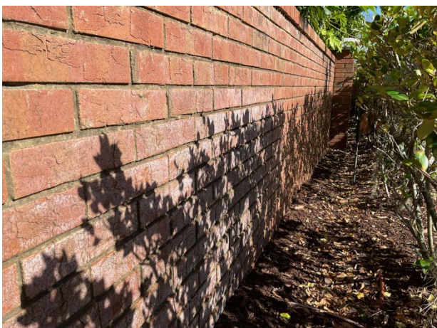
Wall efflorescence at Capri at La Vina
